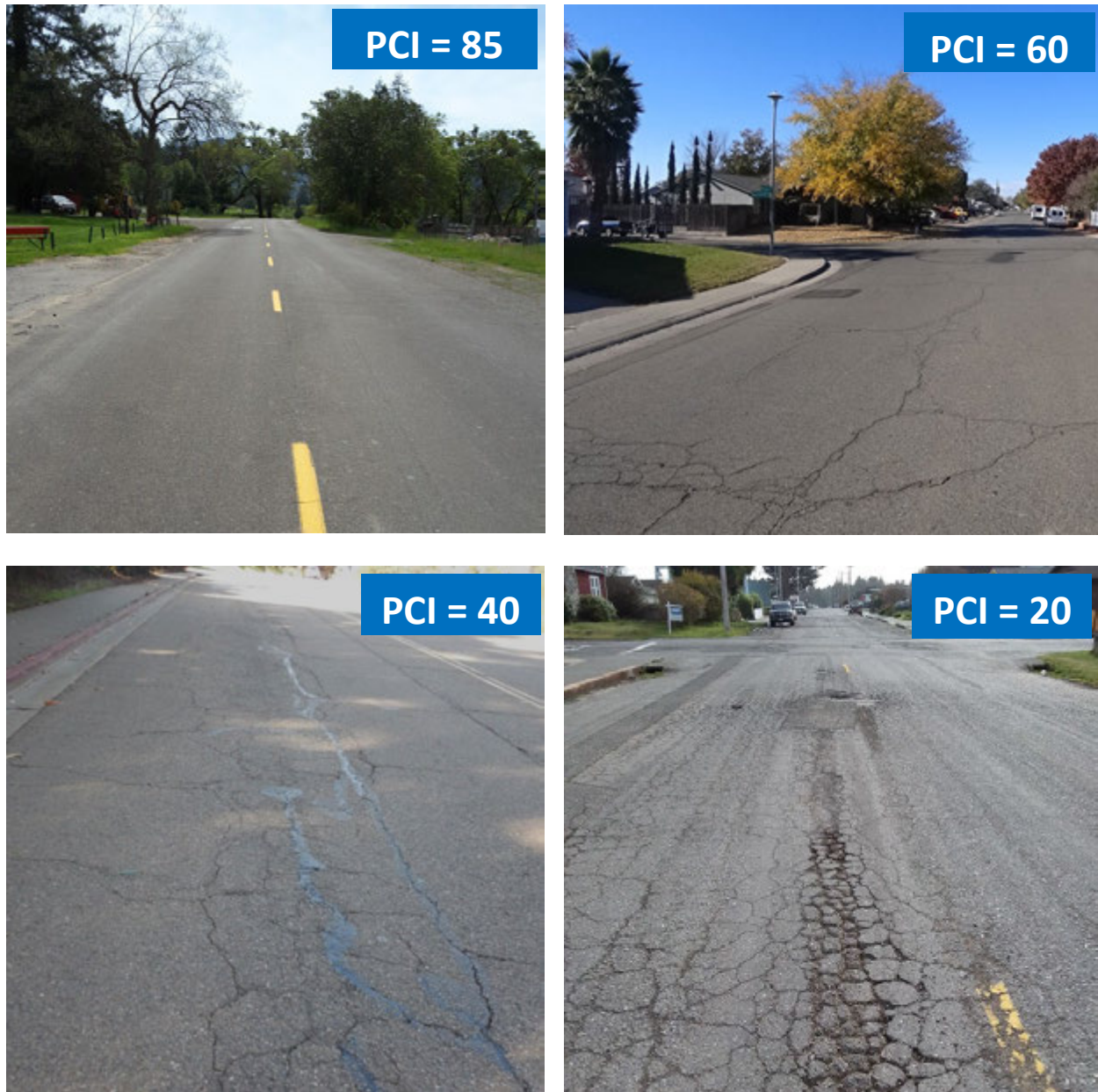
Figure 2. Examples of Streets with Different PCIs
