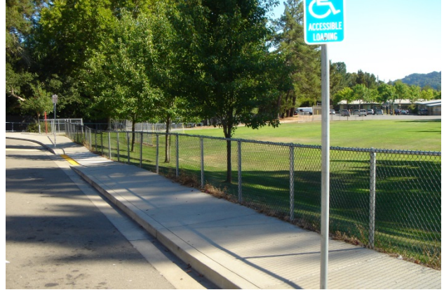
Curb Tight Sidewalk
