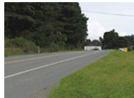
Shoulder Widening, Before (Top) & After (Bottom)
