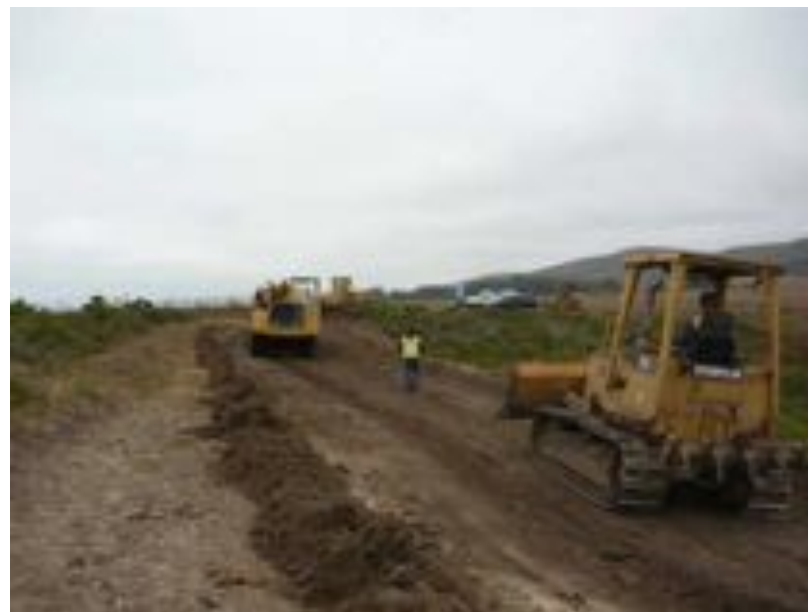
Base rock trail under construction.
