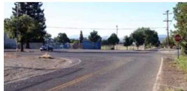
C. The intersection of Airport Road and Howard Street is a large expanse of undefined asphalt and gravel.
