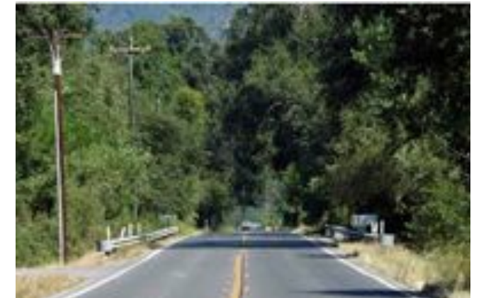
Hwy 162 bridge crossing Mill Creek has narrow shoulders.
