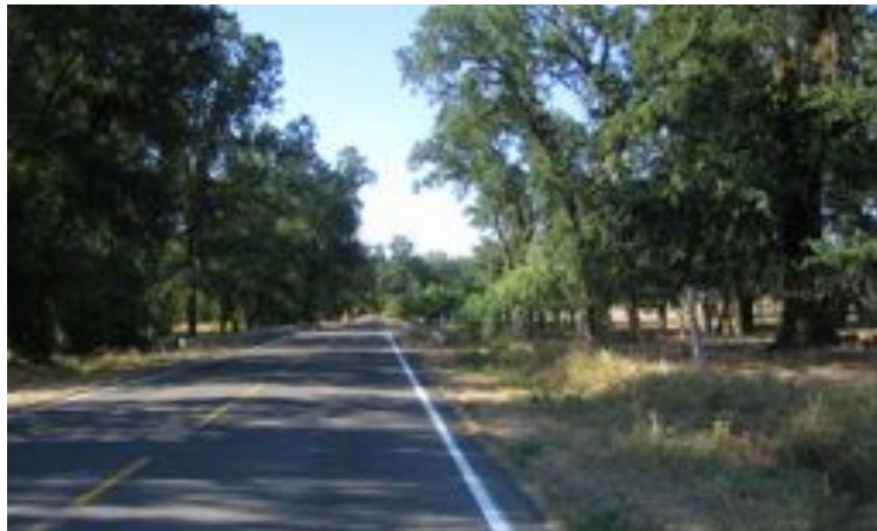
Fairbanks Road (looking east).
